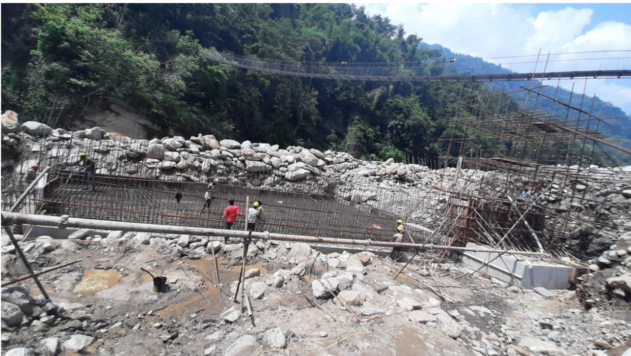
Figure 6: Bar placing and formworks installation works on undersluice bay bottom slab.
