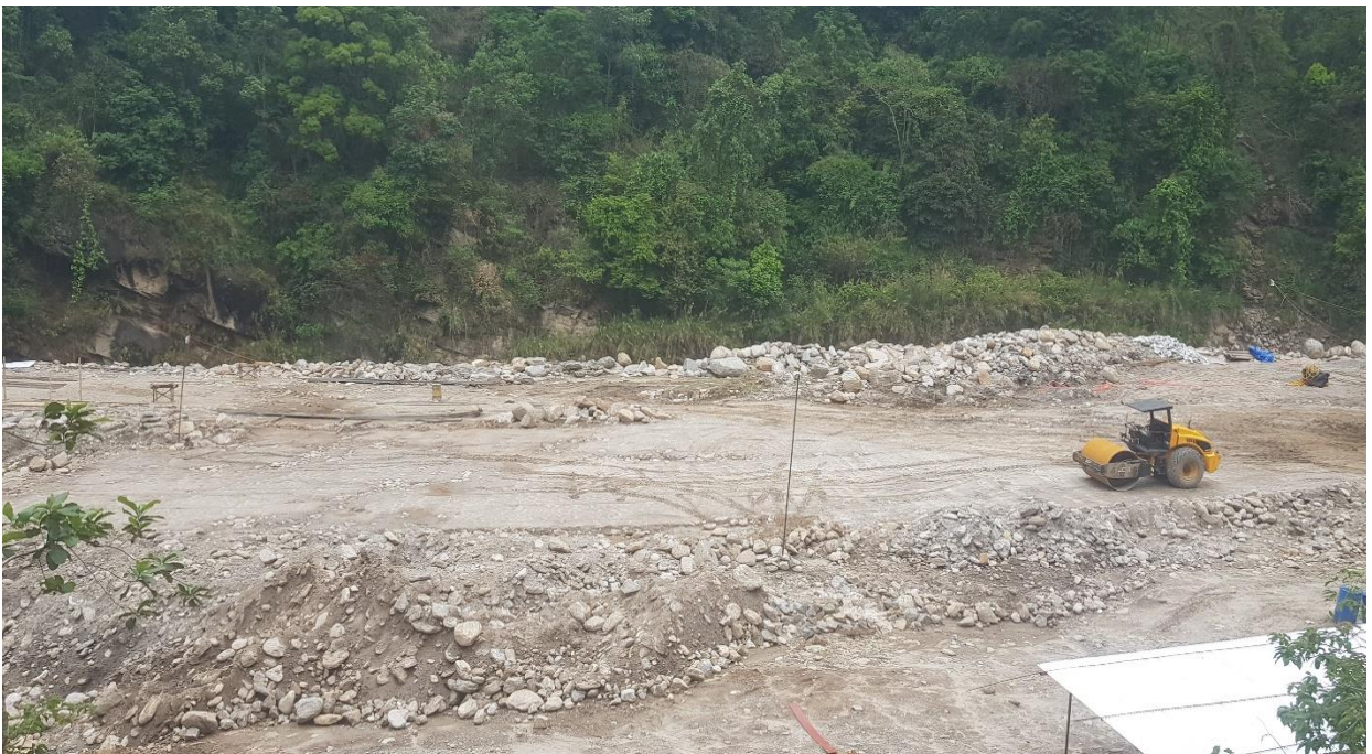
Figure 8: Earthwork in filling and compaction using roller around desander area.
