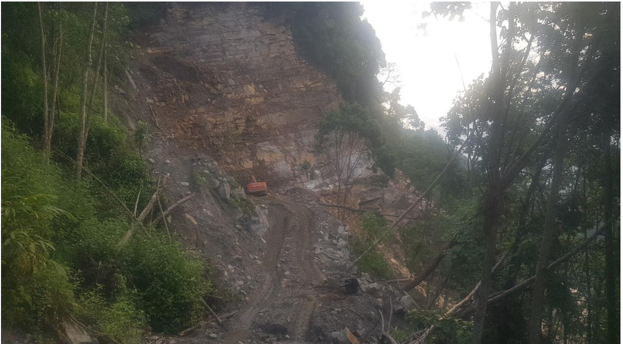
Figure 18: Track opening work and road widening for waterway at rocky area
