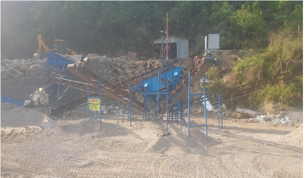
Figure 23: Crusher Plant in operation.
