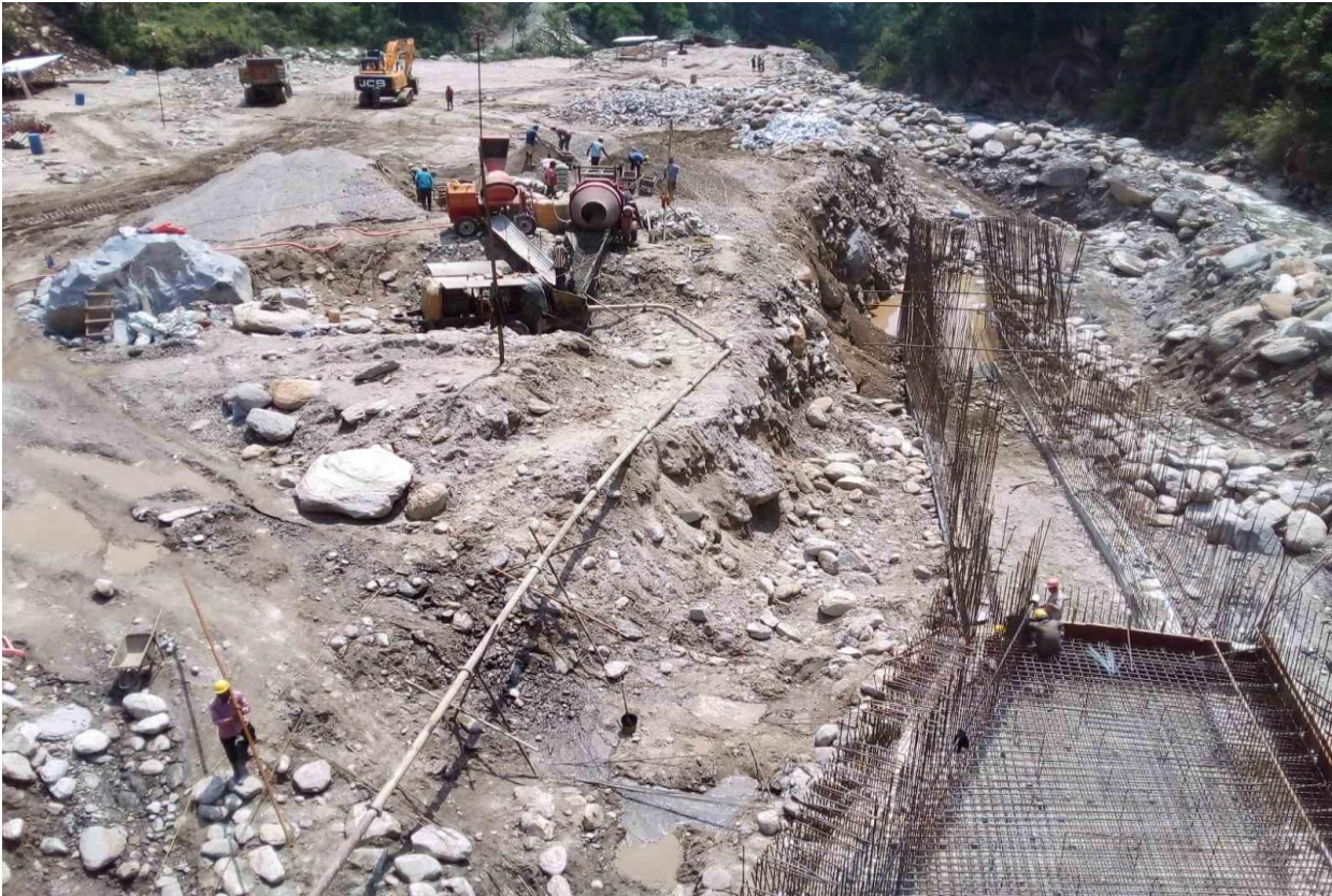
Figure 5: Backfilling work below undersluice slab.
