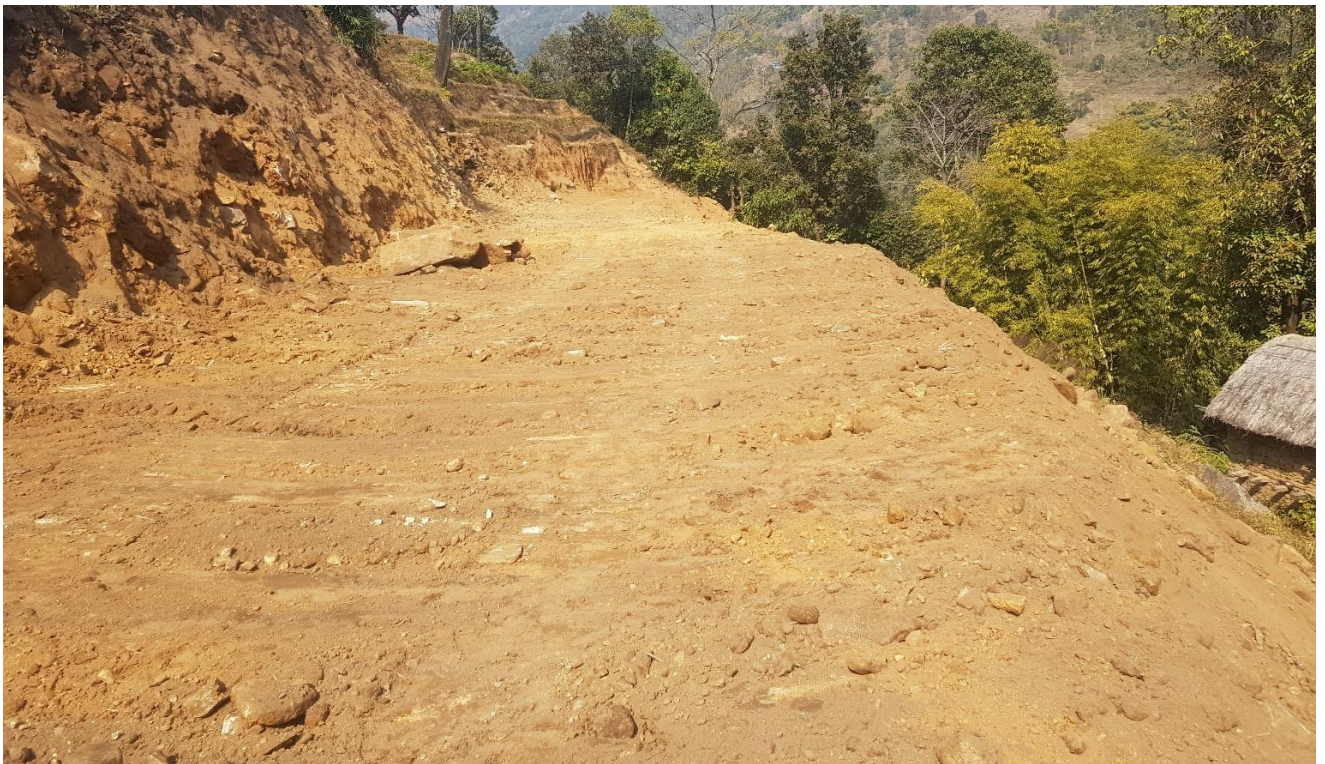
Figure 22: Road Widening for Headrace Pipeline Alignment
