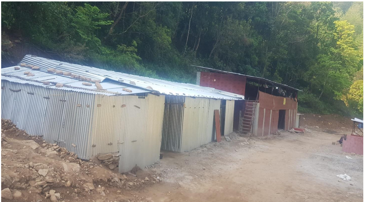
Figure 14: Labour camp and store at headworks
