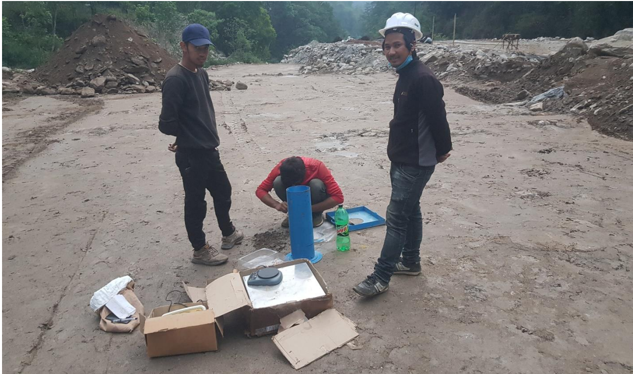
Figure 9: Compaction Testing In desander area.
