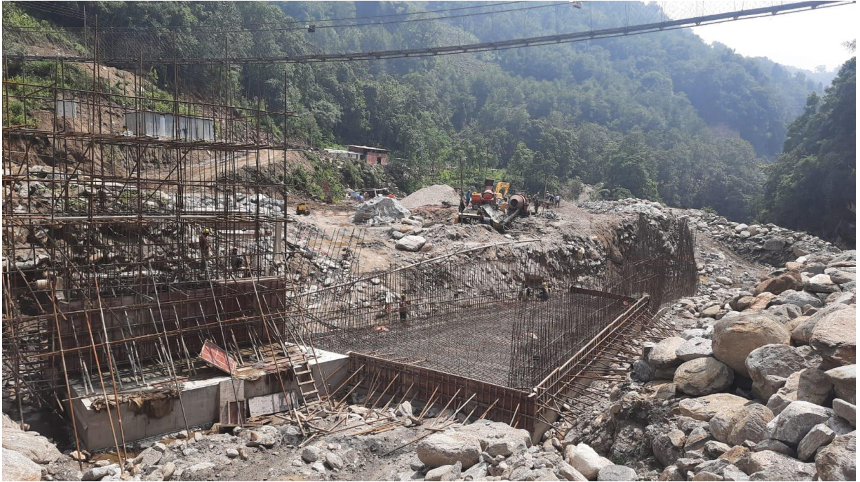
Figure 1: Undersluice, guidewall and intake construction works.
