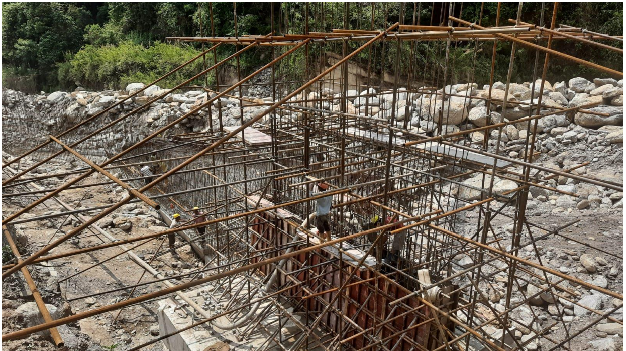
Figure 2: Slab and shear wall concreting on guide wall
