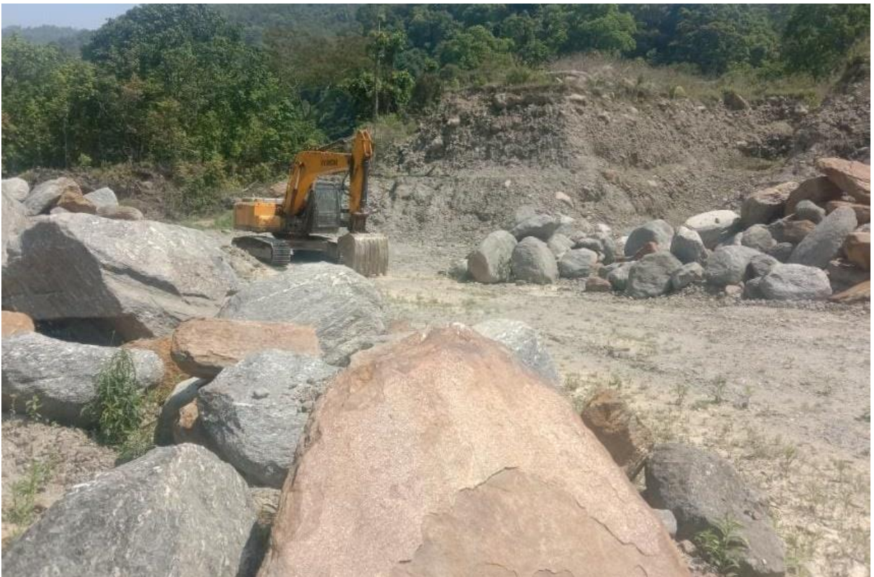
Figure 24: Excavation for Powerhouse Structures.
