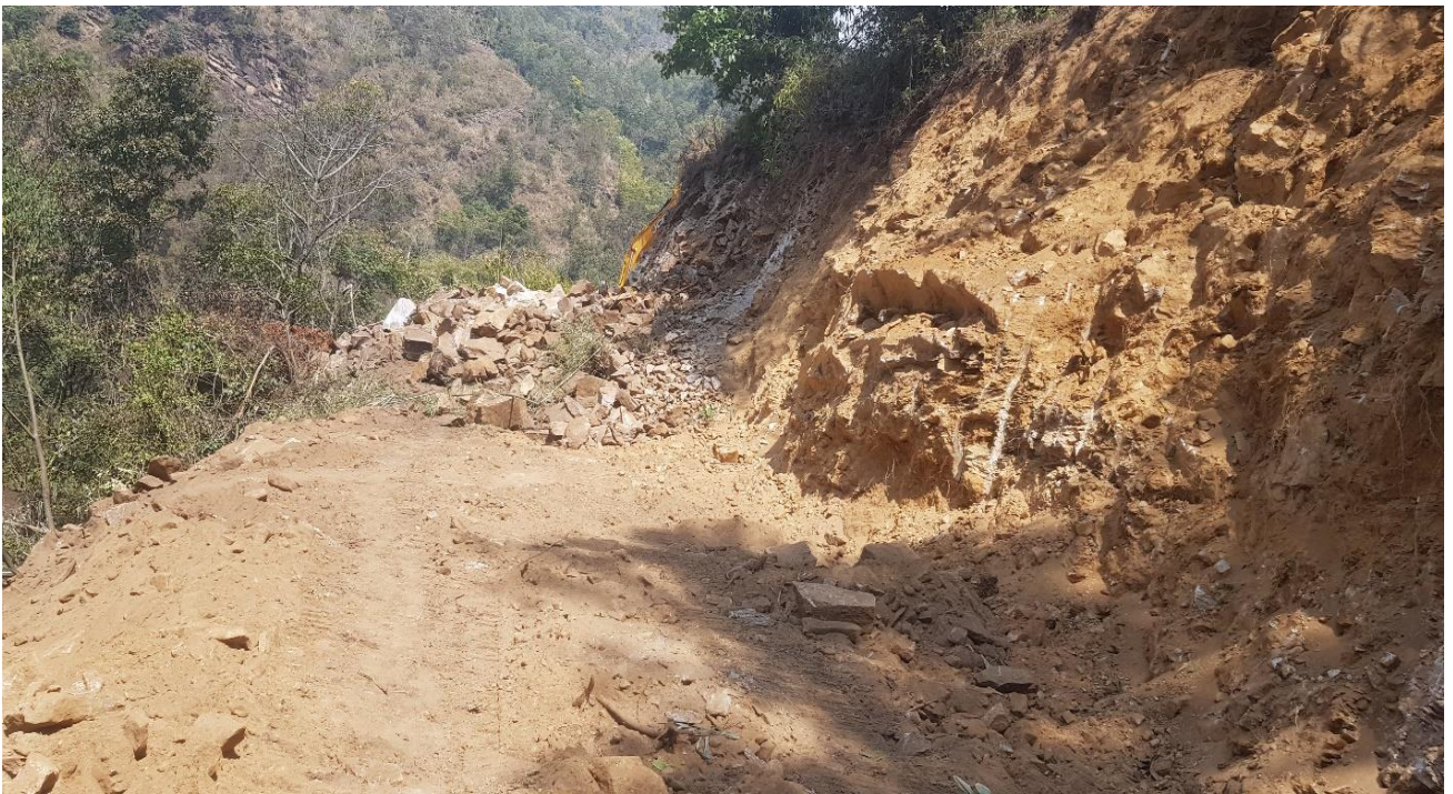
Figure 20: Road Widening for pipeline alignment.
