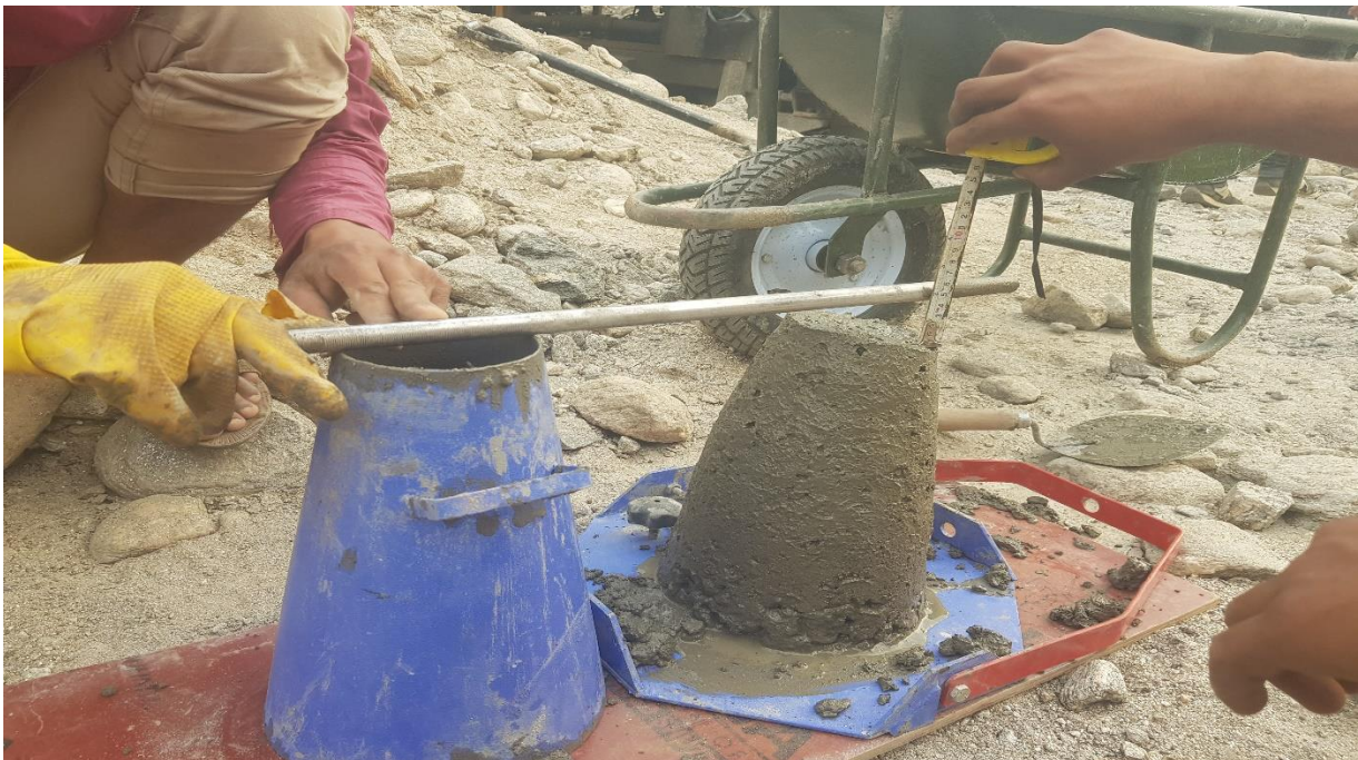
Figure 10: In- site quality control of concrete work.
