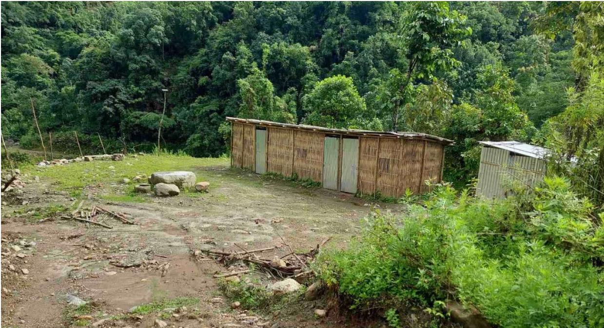
Figure 15: Labour camp at powerhouse
