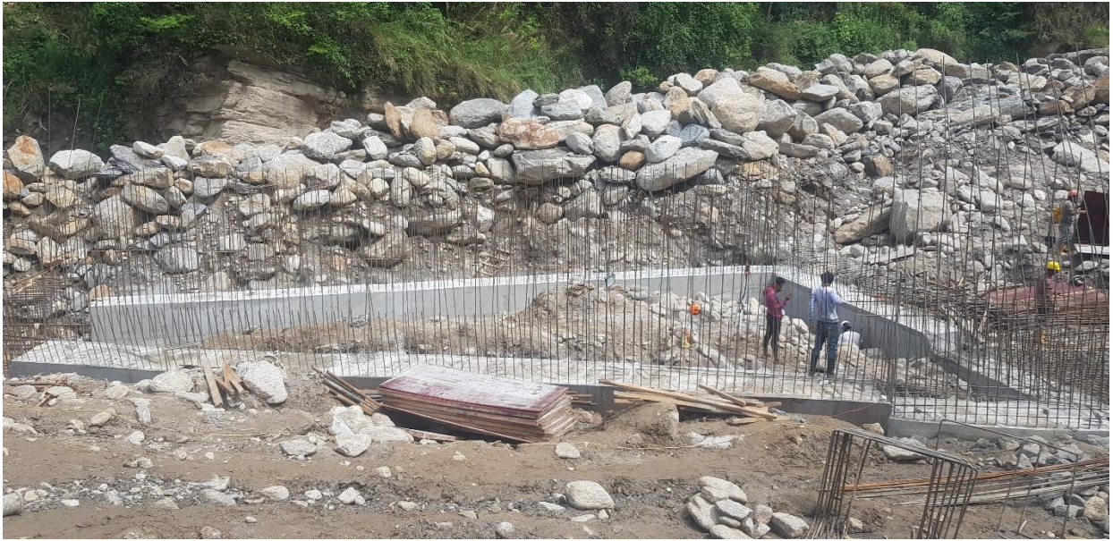
Figure 3: Cutoff Concreting work undersluice upstream bay.
