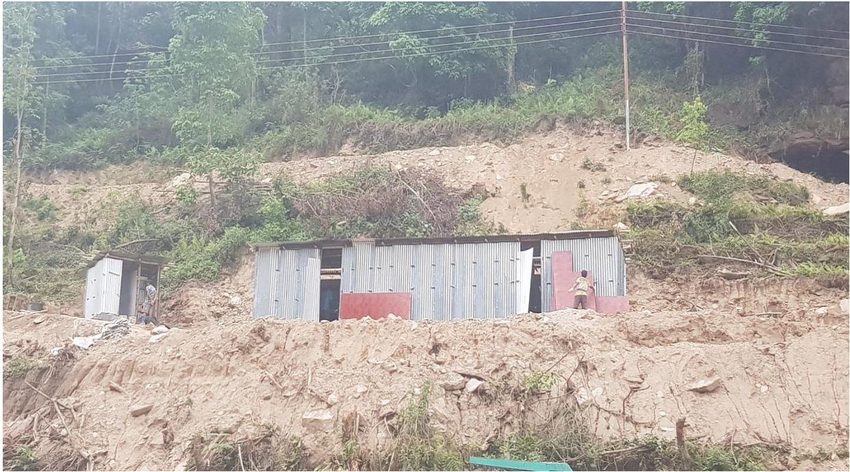
Figure 13: Labour camp headworks
