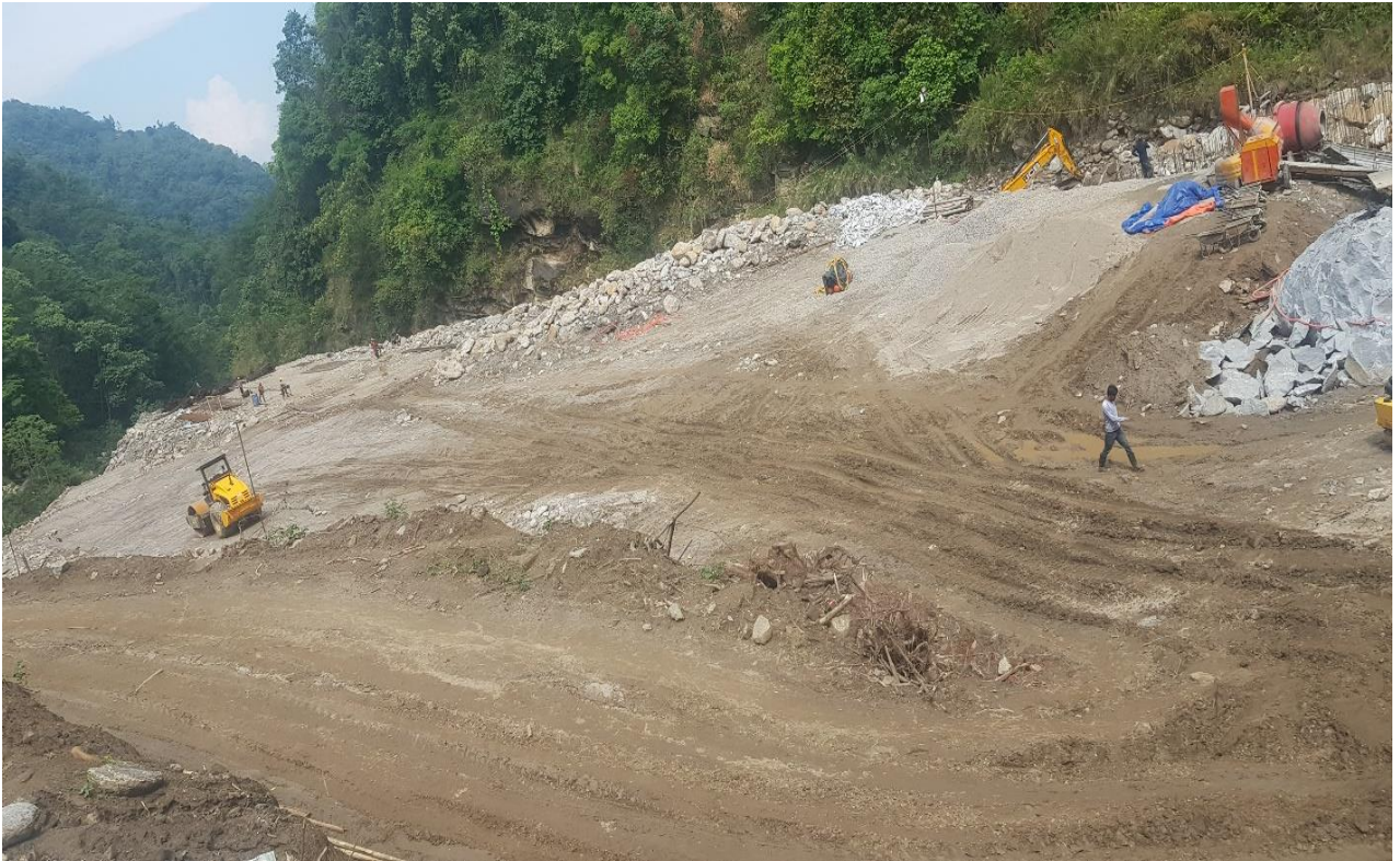
Figure 7: Gravel trap and desander inlet base preparation
