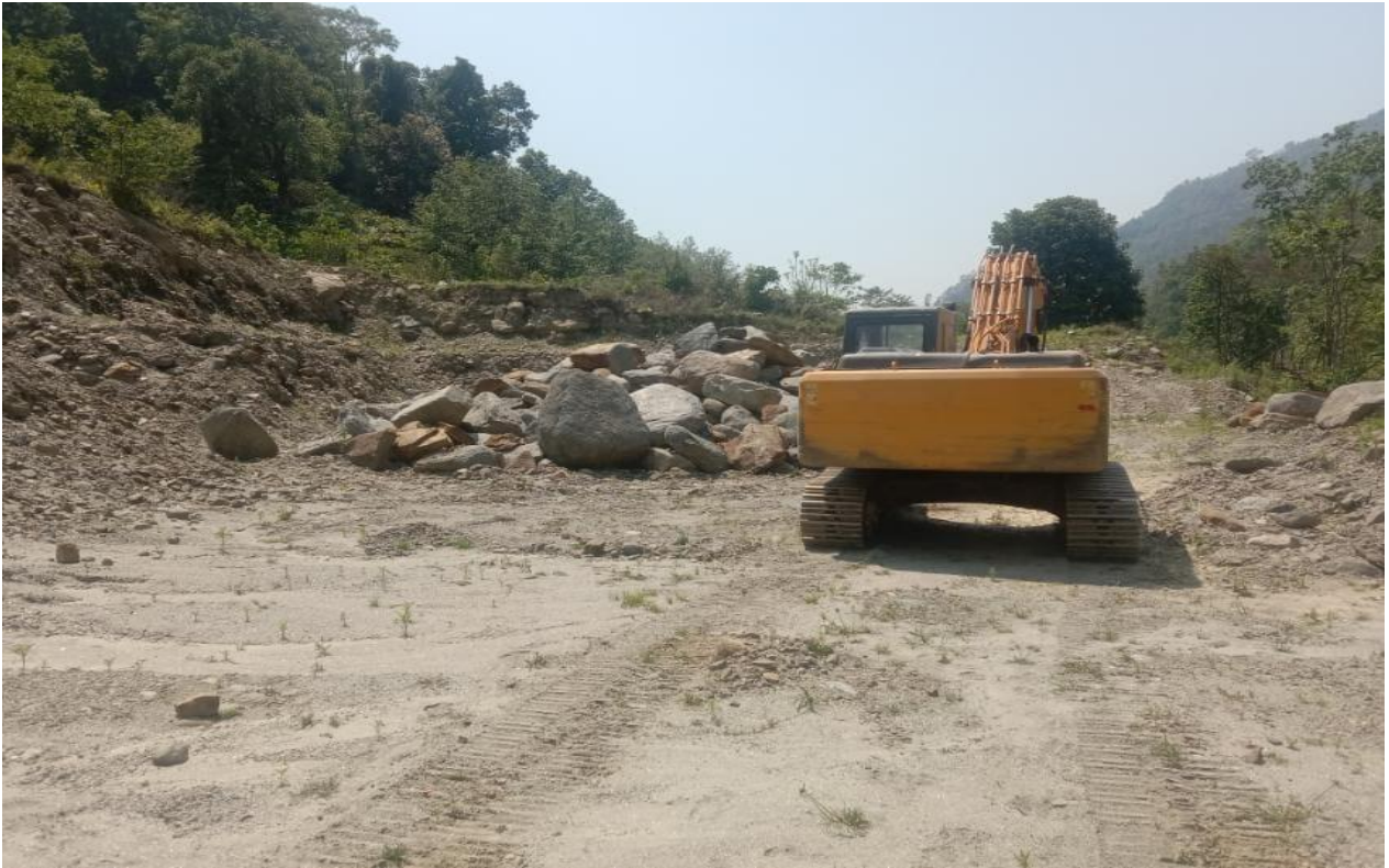
Figure 25: Excavation for Powerhouse Structures
