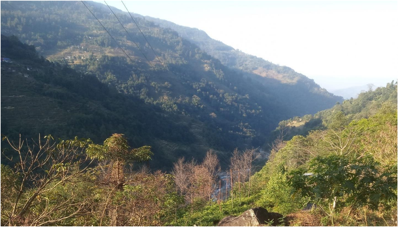
Figure 17: 11 KV Transmission Line for construction power
