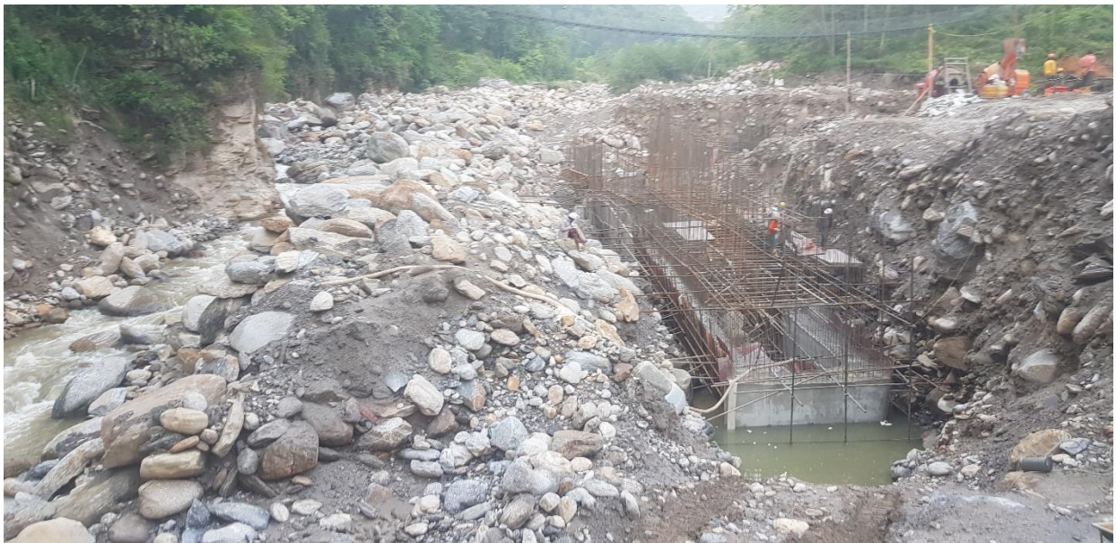
Figure 4: Cutoff Concreting work undersluice downstream.
